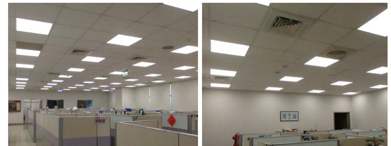
▲ Replacement of LED lighting fixtures in offices and walkways
